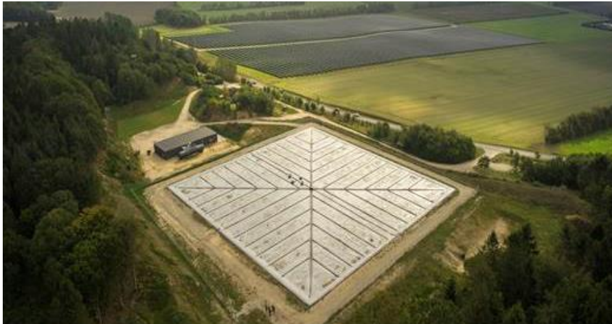
Figure 31 – PTES in Dronninglund, Denmark (Dronninglund Fjernvarme).
