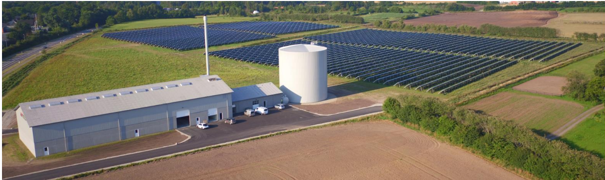
Figure 29 – TTES of 3,000 m 3 in Hjallerup, Denmark in connection to a solar field of 21,500 m 2 and a straw boiler of 1.8 MW th (Hjallerup Fjernvarme).
